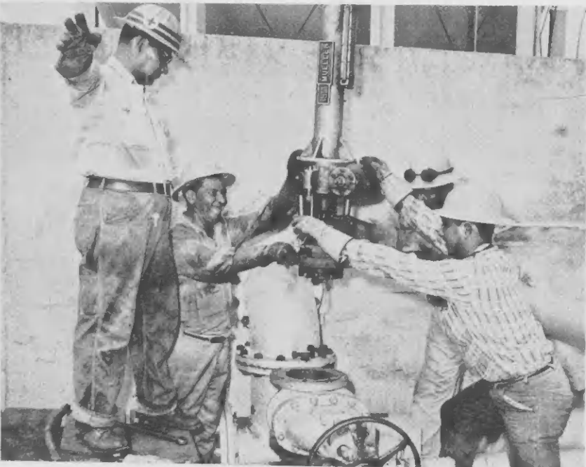
SOON AFTER his suggestion was accepted, Mechanical Department craftsmen began "hot tapping" the kerosine production line, left. PRONTO DESPUES cu su sugerencia a worde aceptá, hendenan di Mechanical Department a cuminsa cu « trabao di "hot tap" ariba e linja di kerosine, robez.
